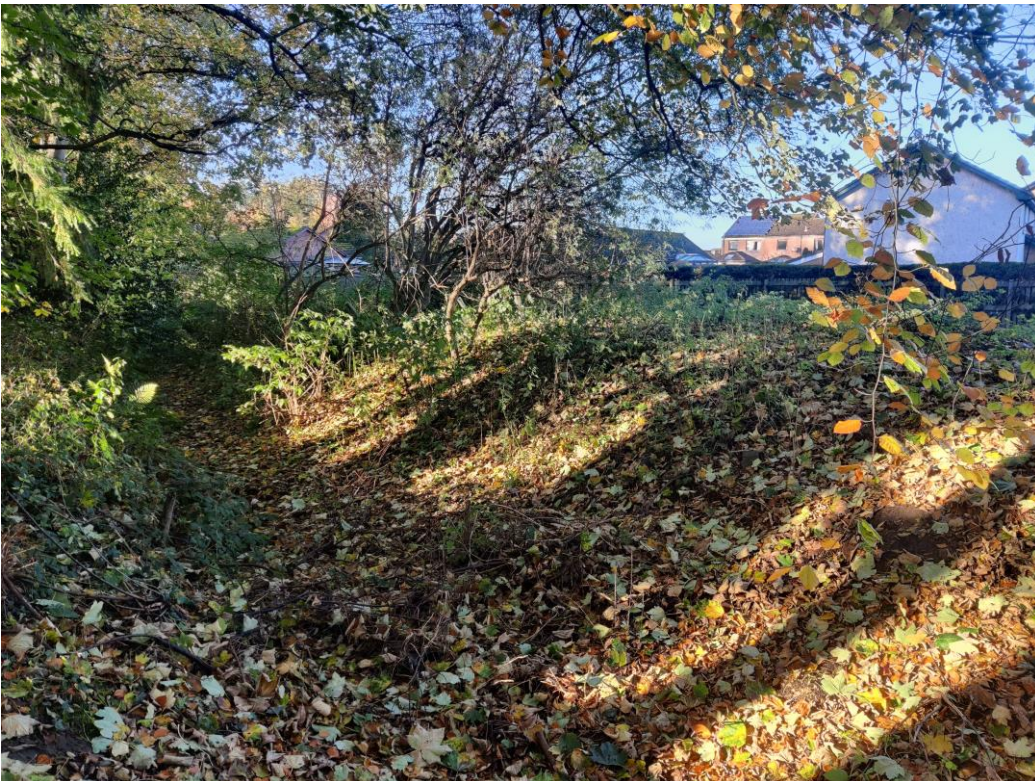
Photo 2: Photo of the land drain
